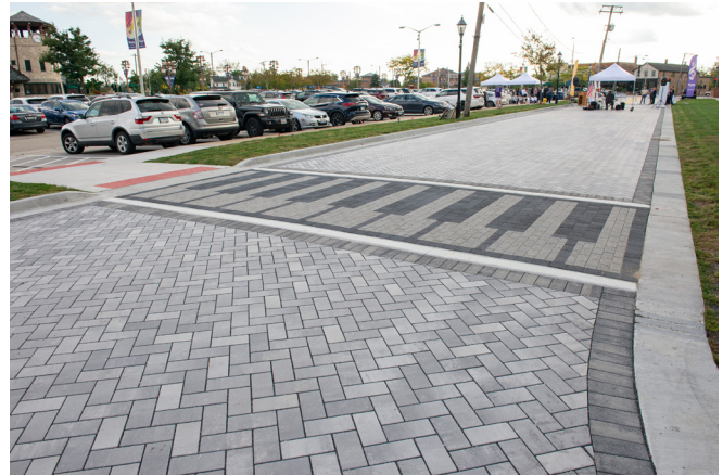
The MWRD joined Tinley Park to fund the installation of 16,500 square feet of permeable pavers arranged to allow water to flow through the gravel joint material and into an aggregate base to reduce up to 69,000 gallons of stormwater from running off. The paver project is part of a larger Harmony Square development.
